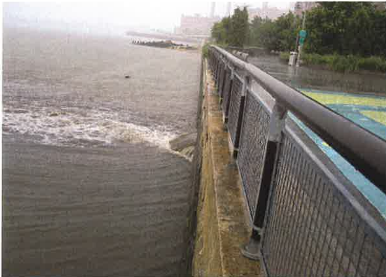
CSO outflow at Stuyvesant Cove Park, one of hundreds around the city Photo: Jamie Paquette, Solar1
