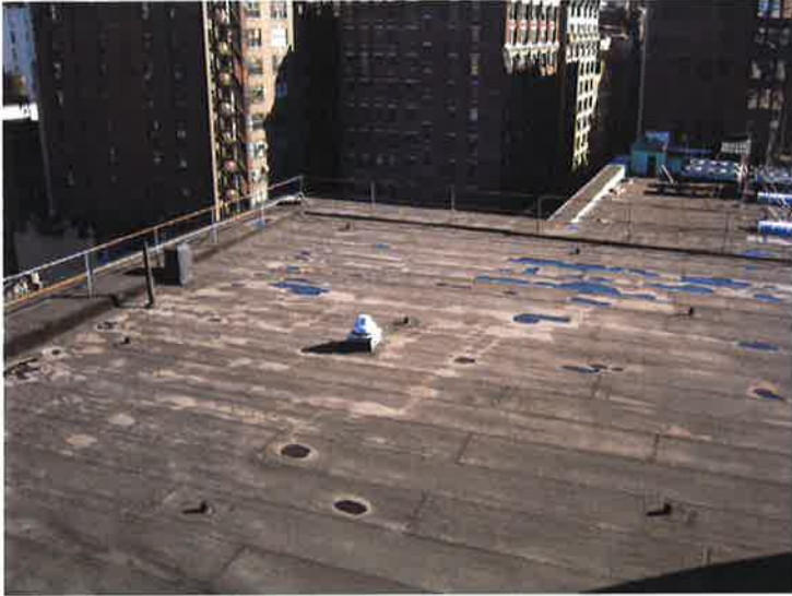
Roof terrace at 641 Avenue of the Americas, before green roof installation
