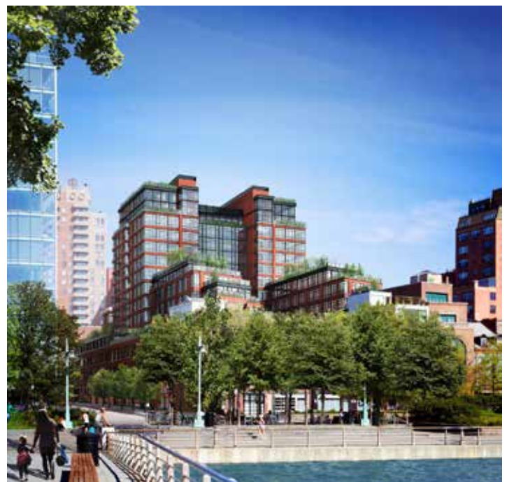
150 Charles Street under construction, June 2015.
